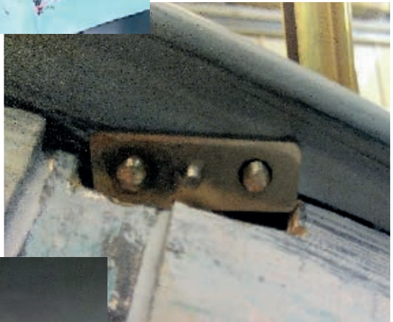
The fixing plate showing the central fixing screw
